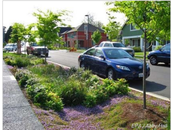
Seattle’s SEA Street (Street Edge Alternatives) project includes bioswales and permeable pavement.
