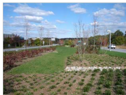
Highway divider strip before and after the retrofit of an infiltration swale.
