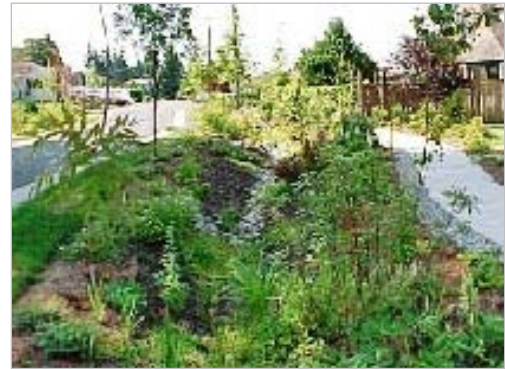
Swale in the middle of Vancouver's Crown Street pilot project. Credit: Vancouver Dept. of Eng.
