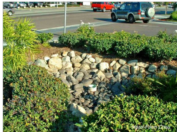
Infiltration swale for a supermarket parking lot. 7676 Firestone Blvd., Downey, CA.
