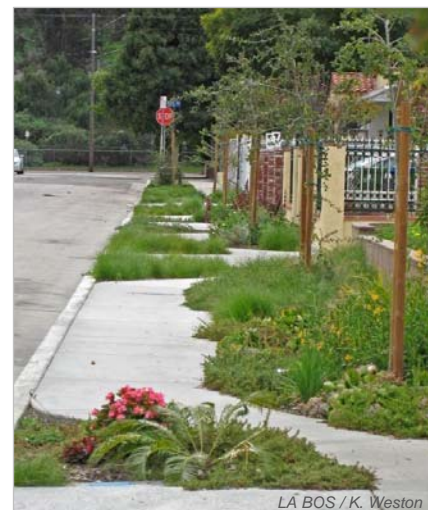
Oros Street after its "green street" reconstruction (Los Angeles)
