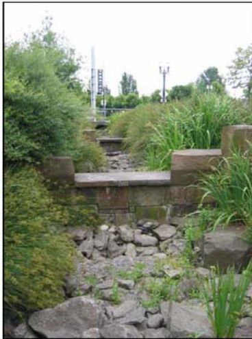
A rain garden manages runoff from impervious surfaces such as roofs and paved areas.
