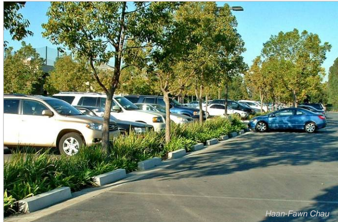
A vegetated swale with curb cuts collects runoff at the RioHondo Golf Course in Downey, CA.
