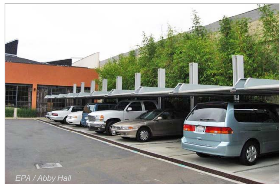
Stacking cars reduces the need for impervious parking lots at this business in Emeryville.
