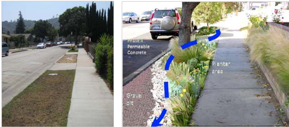
Current view of Riverdale Ave. (left) and design concept for Riverdale green street retrofit (right).
