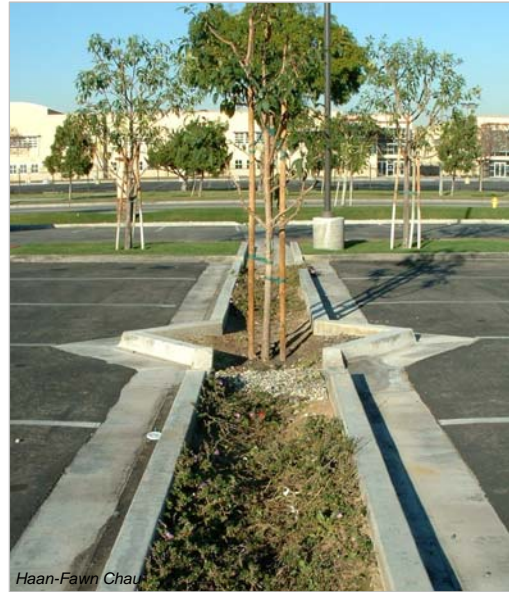
Vegetated swale with curb cuts at a shopping center. 8500 Firestone Blvd., Downey, CA.
